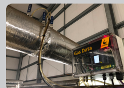
Gas Flow Monitoring
